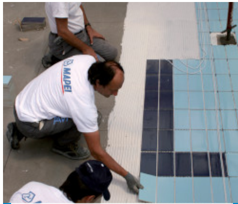
Laying ceramic tiles on Mapelastic in a swimming pool
