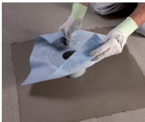
Application of Drain Vertical on Mapelastic
