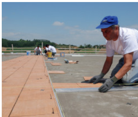
Installing ceramic with Kerabond + Isolastic
