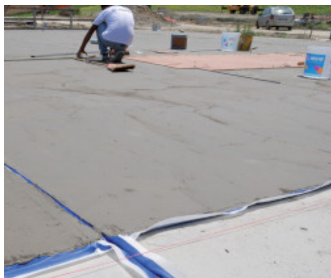
Waterproofing screeds with Mapelastic and Mapeband
