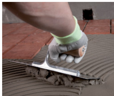
Laying Granirapid on a terrace waterproofed with Mapelastic
