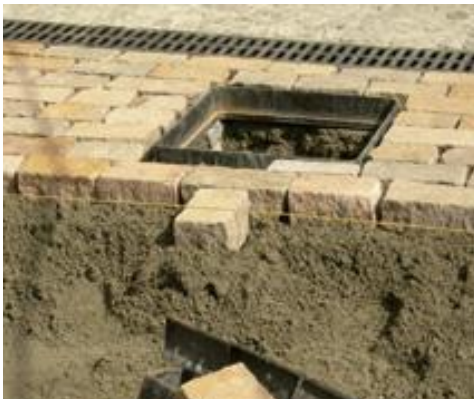
Mapestone TFB 60 mixed to a "no-slump" consistency
