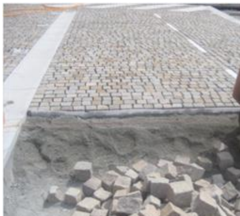
An example of an expansion joint
