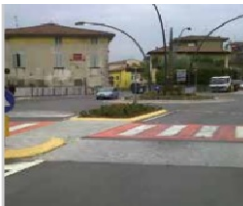
An example of a road hump at a pedestrian crossing
