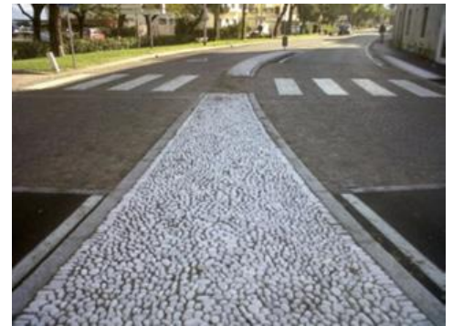
An example of a road with a central reservation in cobblestones
